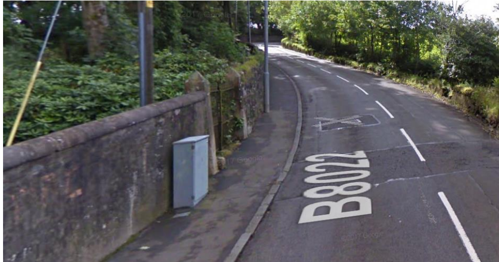
Illus 29: W boundary wall showing the harled brick and concrete coping construction. Note the service drive gate (Author)
