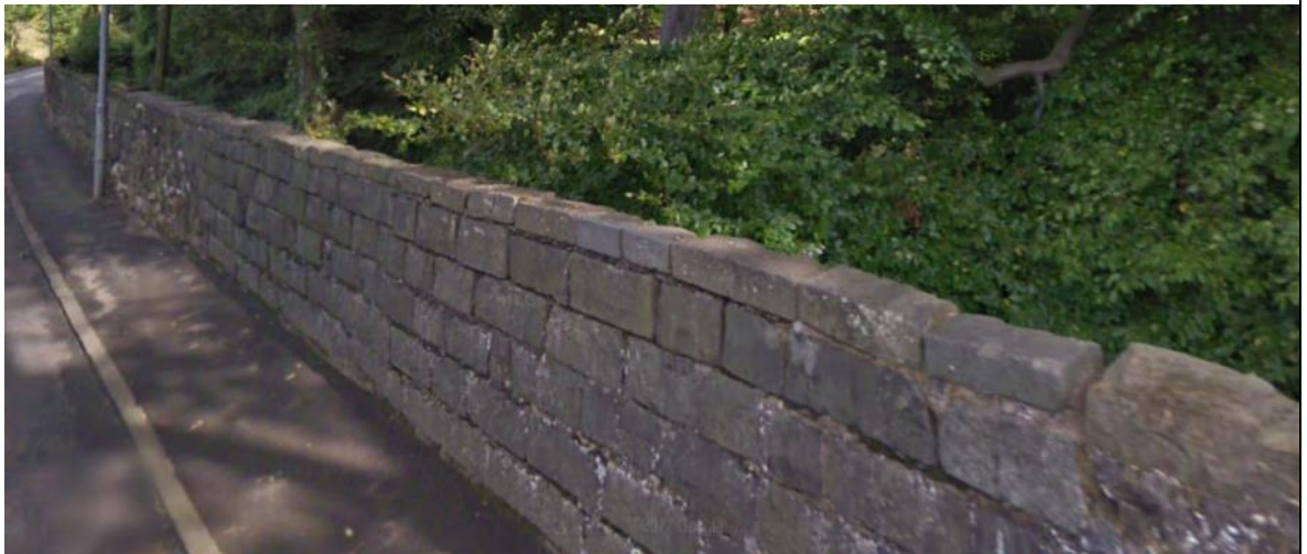
Illus 30 : W boundary wall showing the large rectangular stone infill block at the southern section of the wall (Author)
