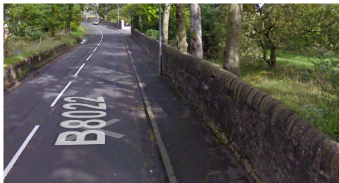
Illus 27: W Boundary wall near the North entrance [white pillar just visible] showing the curved coping stones. (Author)
